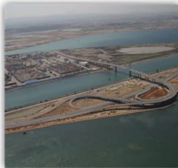
Rades La Goulette Bridge Project
