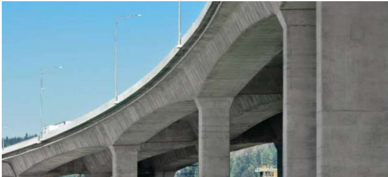
The Port Mann bridge, British Colombia, Canada incorporates Chronolia™
