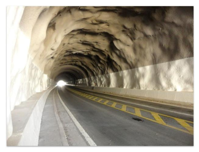
The bidirectional tunnels have two lanes 3,50m wide, a 1,00m central median, two 0,90m sidewalks and New Jersey barriers immersed in the tunnel walls. No lighting was initially provided, as there was no electricity in the area. A recently built transmission line, made possible by the existence of the road, will be used provide energy for tunnel lighting.
