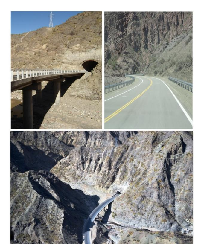
Thanks to a combination of bridges and tunnels and a fairly generous geometric design, the Porto Alegre- Coquimbo Road Corridor crosses the difficult Ischigualasto mountain range in suitable conditions for commercial long distance traffic.
