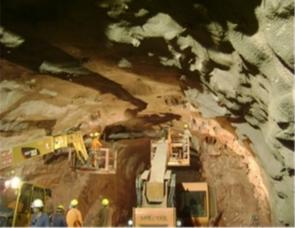
Most tunnels were excavated in formations of poor and very poor rock quality (RMR), with drill and blast methods, where a wide combination of shotcrete reinforced with steel fibres, steel rock bolts and steel ribs was used. The extremely dry climate of the area helps to avoid expensive waterproofing systems.
