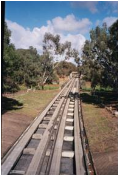
c) O-bahn kerb-guided busway, Adelaide, Australia
