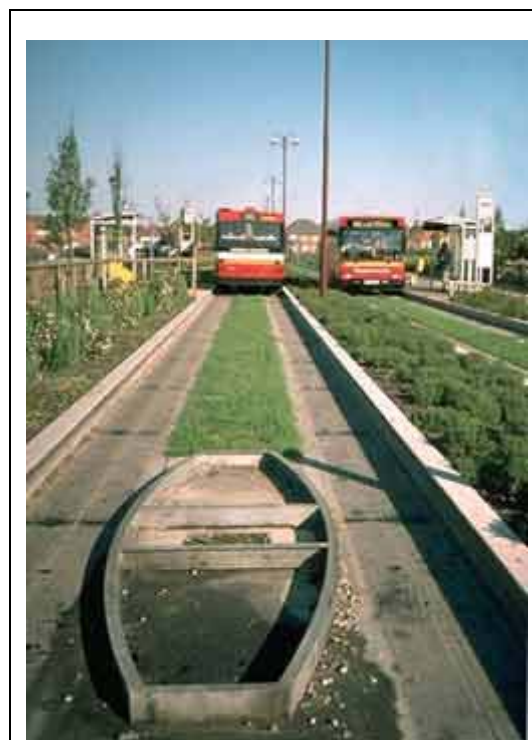
Plate 2 A car trap at a guideway entrance, Ipswich UK
