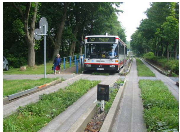
f) Pedestrian crossing, Essen O-Bahn, Germany
