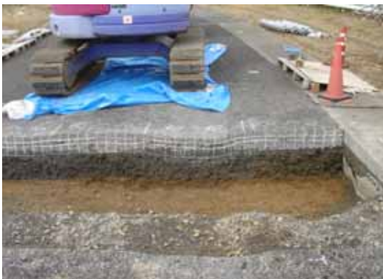
Photograph 1 Damage by softening of the subgrade
