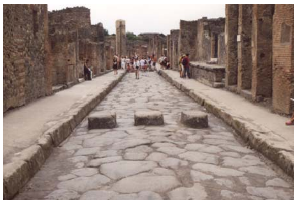
Figure 1: Cobblestone pavement in Pompei (Italy)
