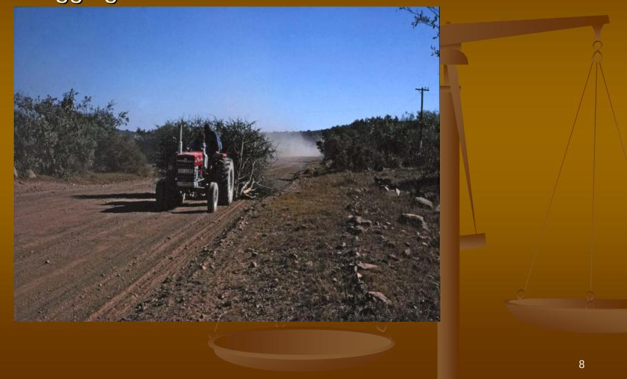
The Spoor Machine was used to improve the sand tracks by making furrows in the heavy sand to assist the drivers to maintain their positions in the tracks, thereby reducing the chances of getting stuck in the sand and also minimizing accidents
