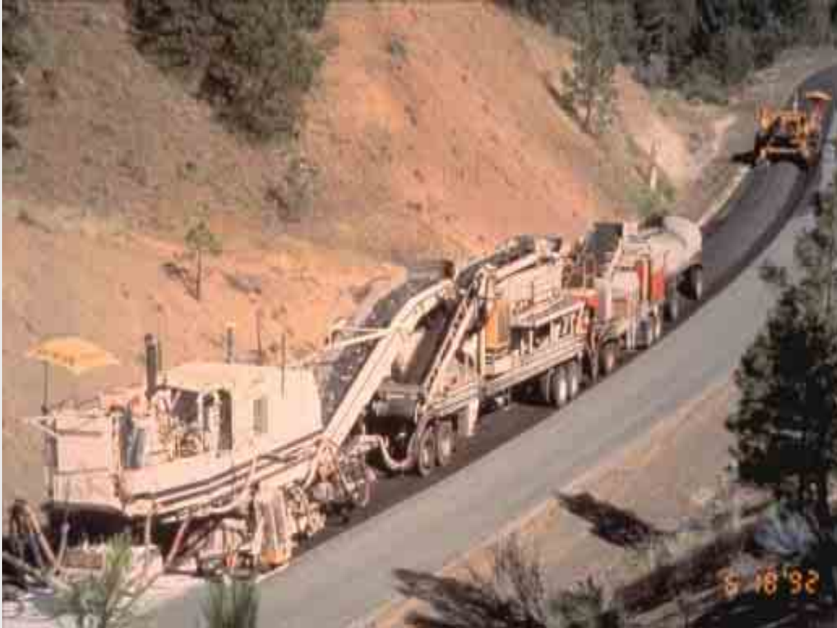
Cold In-Place Recycling
