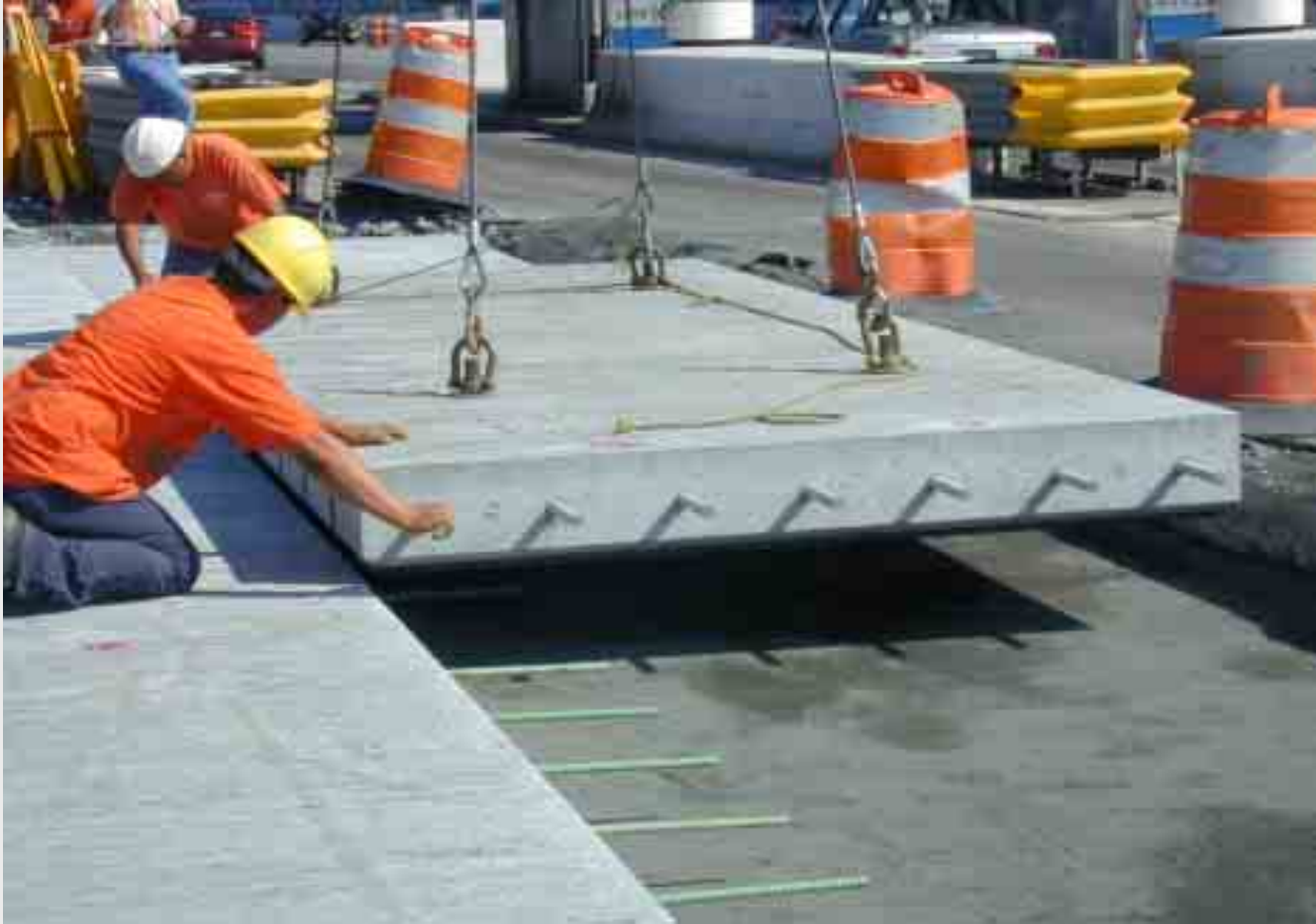
Pre-cast concrete slab replacement
