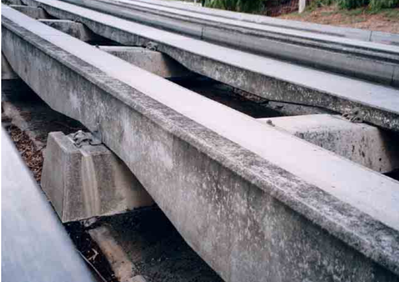
Precast concrete beams and sleepers, Adelaide, Australia
