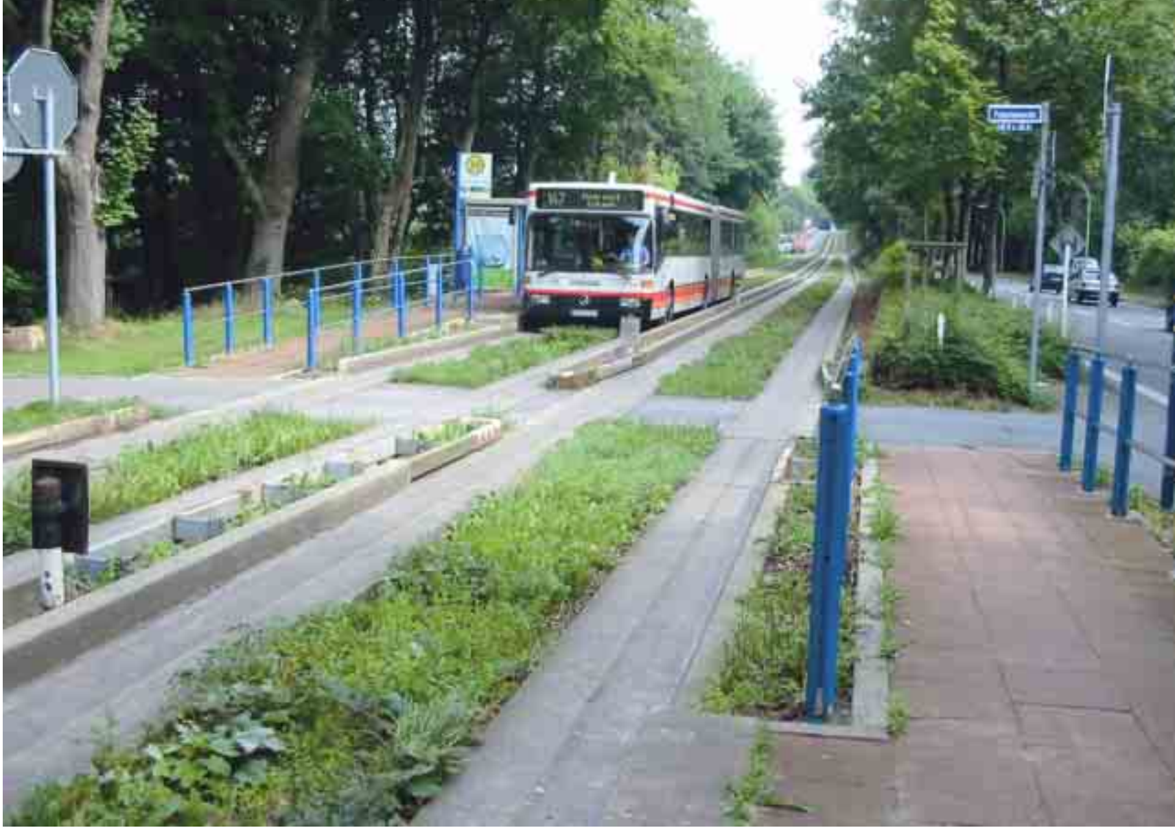
Guideway crossing, Essen, Germany
