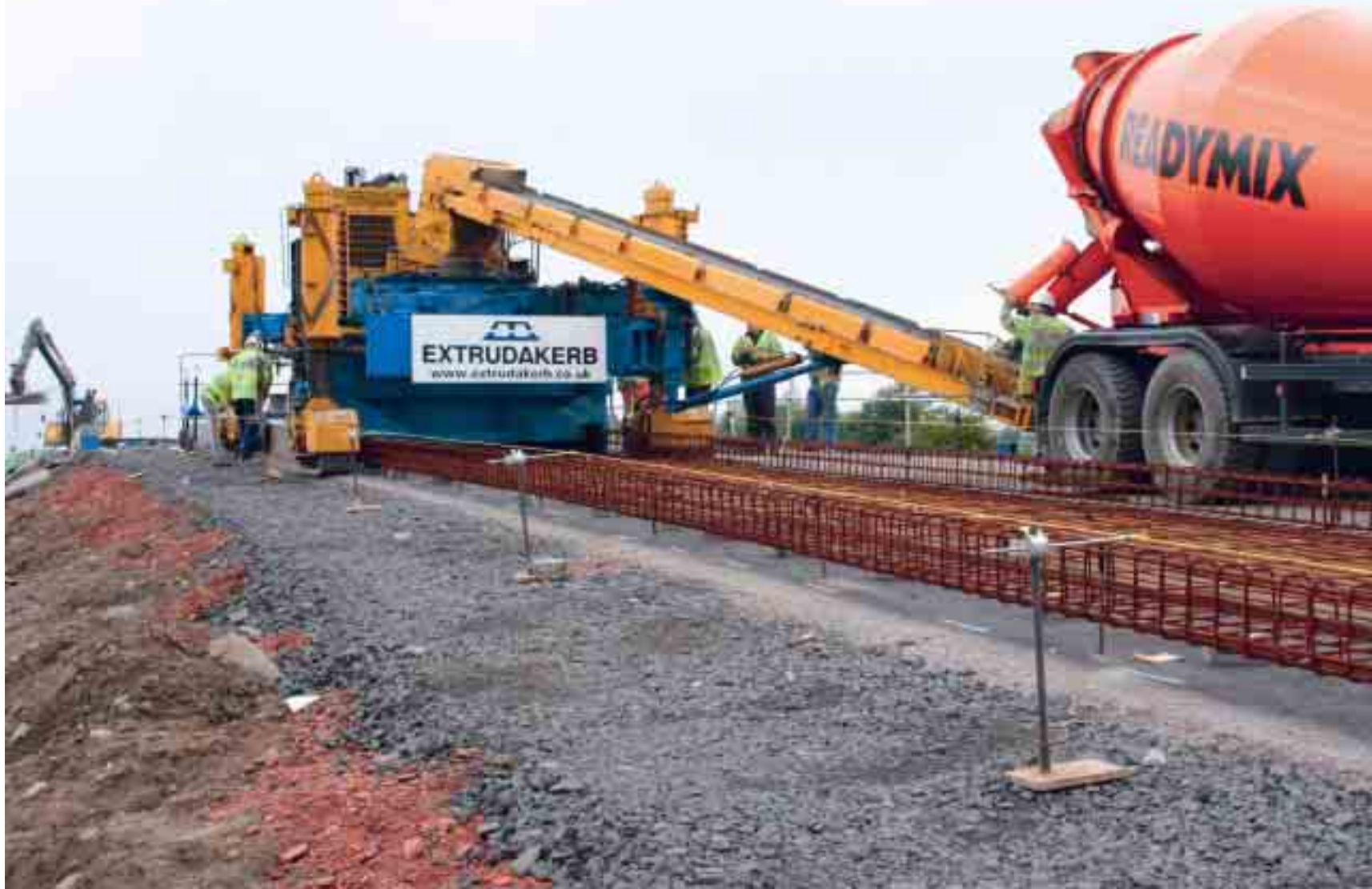
Reinforcement cage anchored into a base slab, Edinburgh, UK
