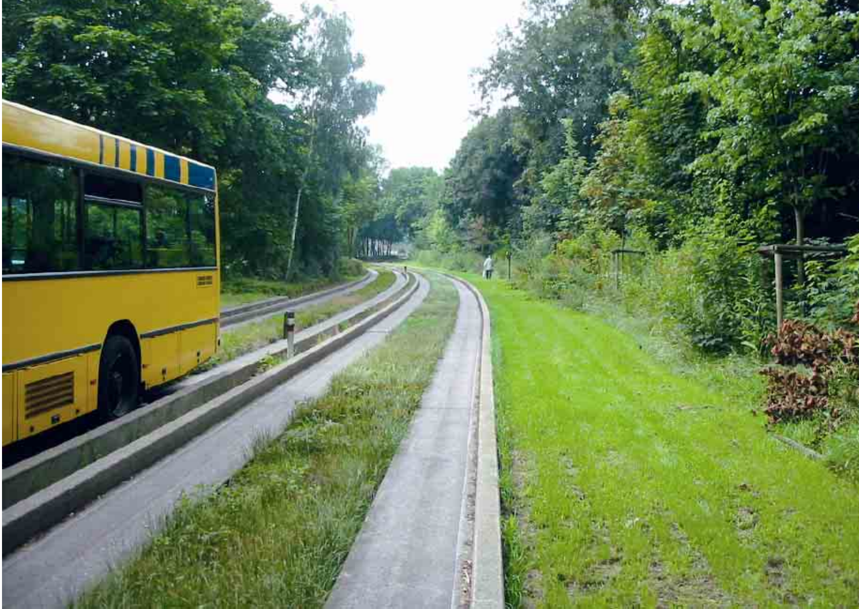
Guideway with central planting and landscaping Essen Germany
