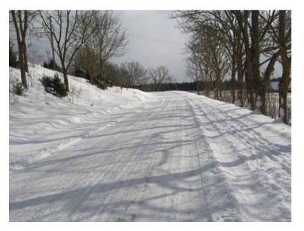
Road surface is allowed to be covered with snow or ice anti-skid treatment only in dangerous places. There may be dry and light snow up to 10 cm or wet thaw snow, sleet or salt-snow mix up to 6 cm.
