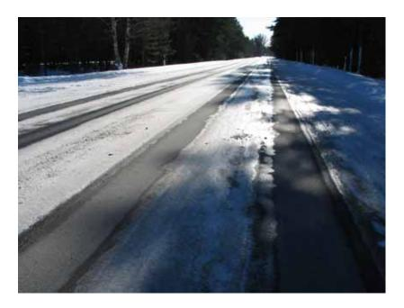
Surface is allowed to be covered with snow or ice, anti-skid treatment is required. There may be dry and light snow up to 5 cm or wet thaw snow, sleet or salt-snow mix up to 3 cm.
