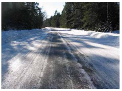
Wheel tracks must be clear. There may be dry and light snow up to 3 cm or wet thaw snow, sleet or salt-snow mix up to 2 cm between wheel tracks  $2^{nd}$  level of maintenance
