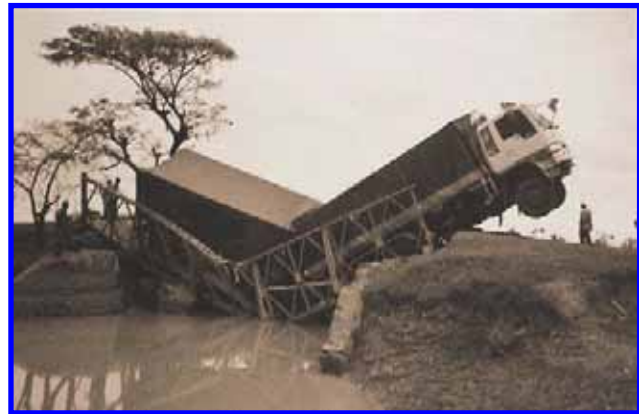
Figure 4 – Overloaded truck damages bridge on a secondary road.
