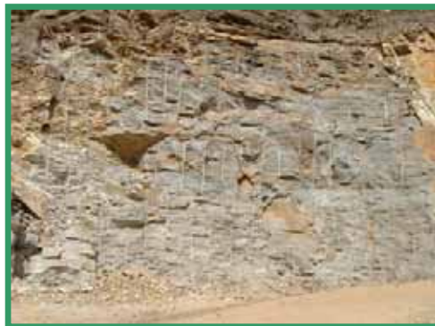
Pictures left: Log barrier and stable slope after controlled blasting
