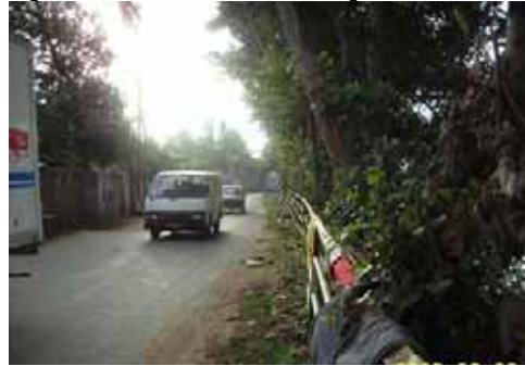
Fig.8 - No LHS side drains throughout the road.
