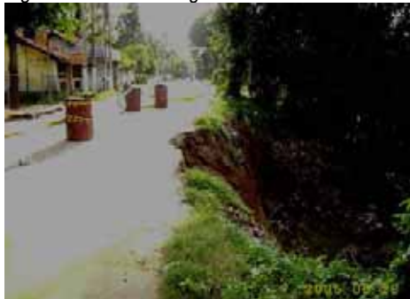
Fig.9 - The diminishing RHS shoulder.
