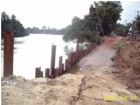
Fig.11 - Row of sheet piles at the apex of the meander "A"
