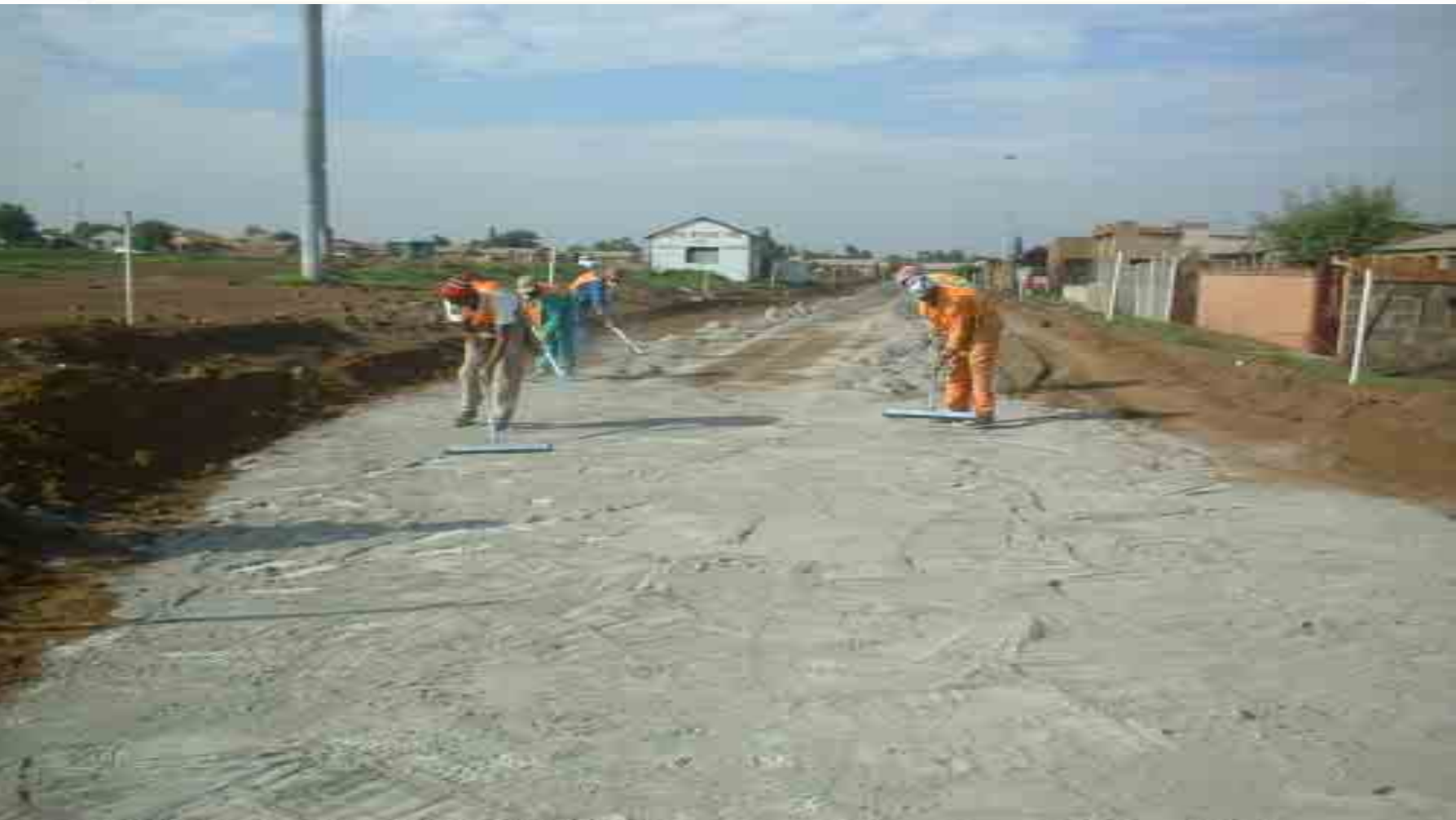
Stabilisation of Base in Pimville
