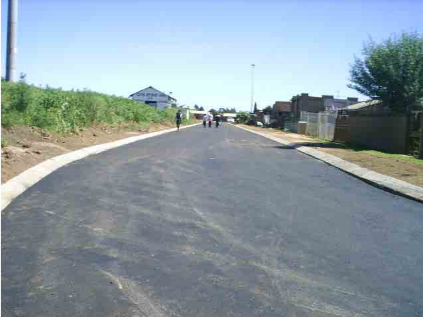
Completed Road in Pimville
