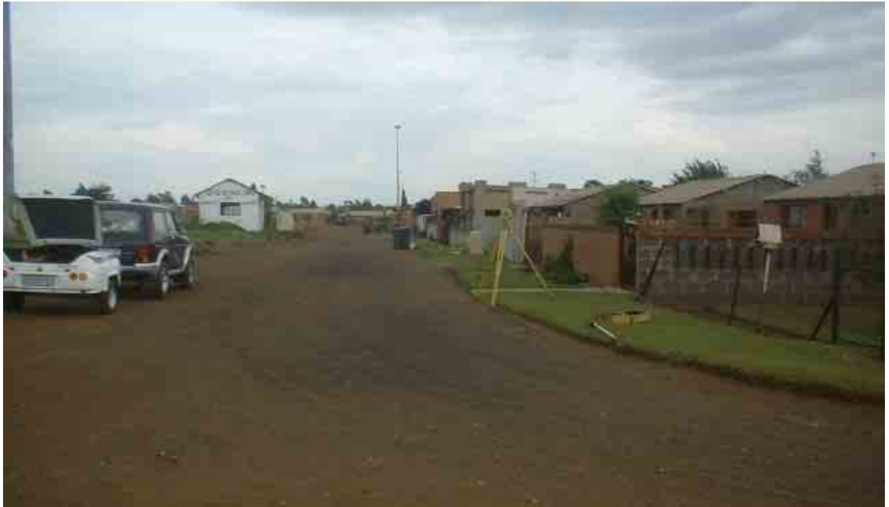
Road being Surveyed in Pimville
