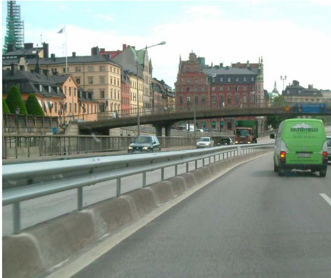
An example of a bad method for separation of traffic directions! The concrete barrier is too low and it has been several vehicles vaulting over it. A steel beam barrier had to be added to get the necessary height.
