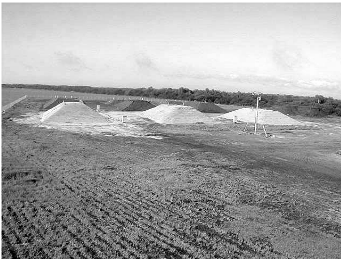
Photo 1 Experiment of test embankment
