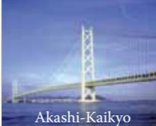
Akashi-Kaikyo                      | Japan   | Akashi Kaikyo Bridge is a steel suspension bridge, which is located on Kobe-Awaji-Naruto Expressway between Honshu island and Shikoku island. It has six traffic lanes. Total length is 3,911 m with span configuration of a centre span 1,991 m and two 960 m outer spans. The centre span length is the longest single span in the world. Bridge girder is a truss type with steel deck. ( <i>picture 3, pp. 30-31</i> ) |
