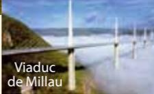
Viaduc de Millau                   | France  | Multi span cable stayed bridges - Span length 342 m; total length 2,460 m - Steel box girder - Built: 2004                                                                                                                                                                                                                                                                                                                 |
