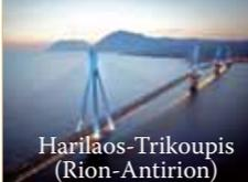
Harilaos-Trikoupis (Rion-Antirion) | Greece  | Harilaos Trikoupis Bridge (ex Rion - Antirion Bridge) links mainland Greece with Peloponnese. The main bridge is a 5-span cable stayed bridge that consists of 3 spans of 560 m and 2 side spans of 286 m. ( <i>picture 2, next page</i> )<br>Composite steel beams - concrete deck<br>Built: 2004                                                                                                                         |
