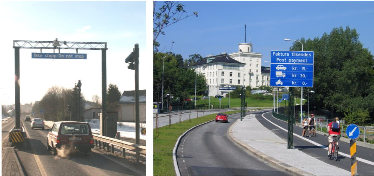
*Figure 8: Fully automated free flow road toll stations in Tønsberg and Bergen*
