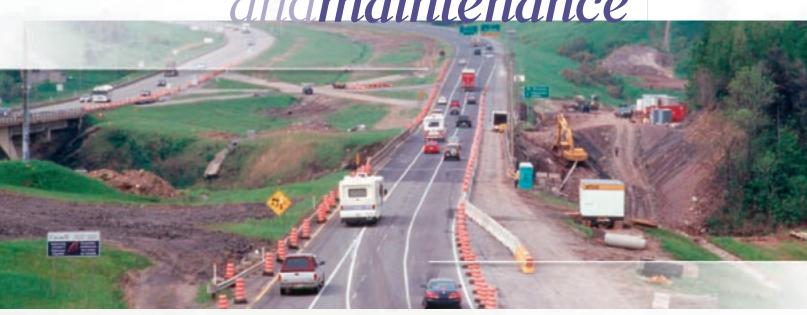
Most of the primary road network was designed over 30 years ago. Since then, the total authorized loads, which have increased by 10% to 40%, are straining and hastening the deterioration of roads and structures. Québec winters, with lengthy periods of heavy frost (to a depth of 1.2 m to 3 m) and daily temperature changes of up to 25 °C, are gradually warping the roads, a situation that is exacerbated during thawing.
