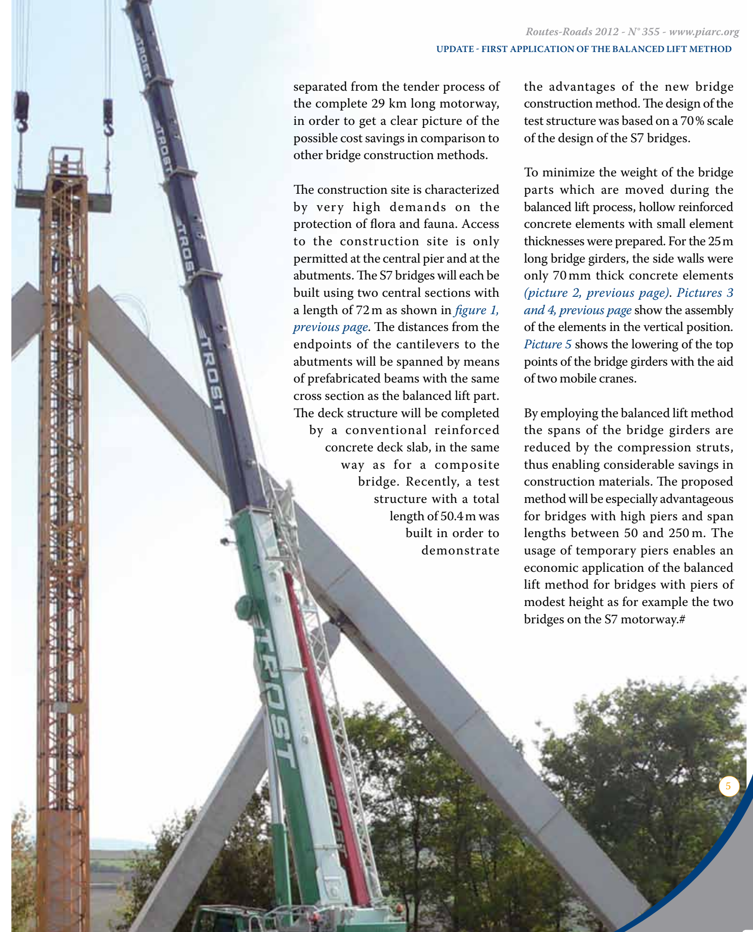
Picture 5 - Lowering of top points of bridge girders with the aid of mobile cranes
