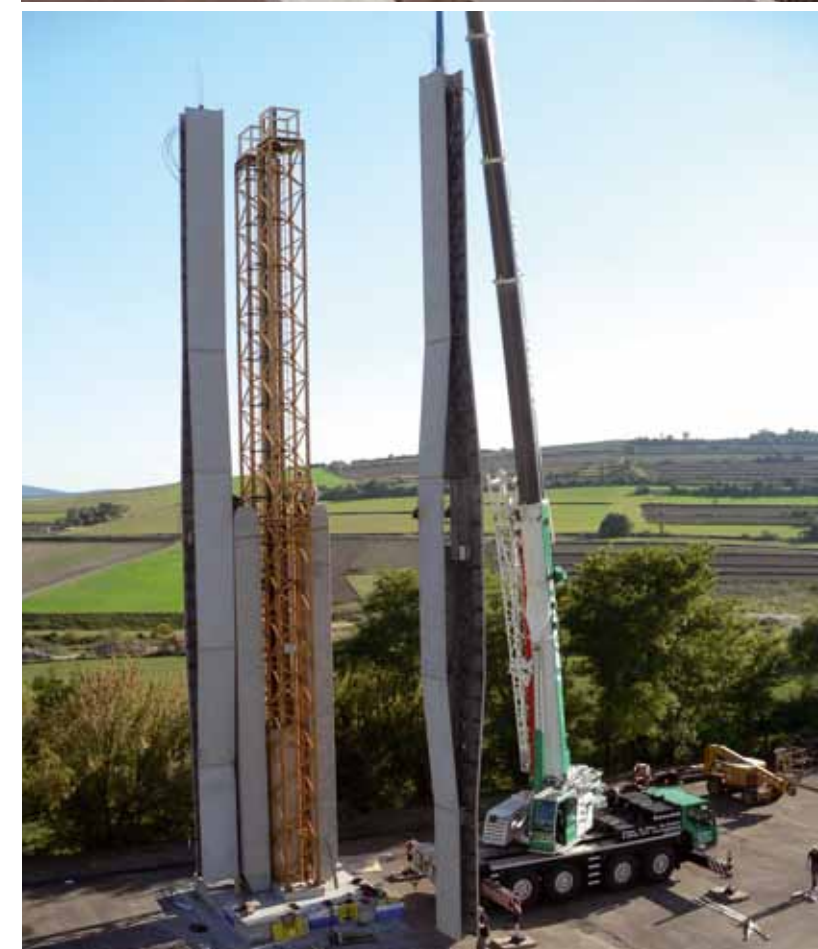
Illustration 1, left page - Bridge structures on the S7 motorway and test structure for the balanced lift method
