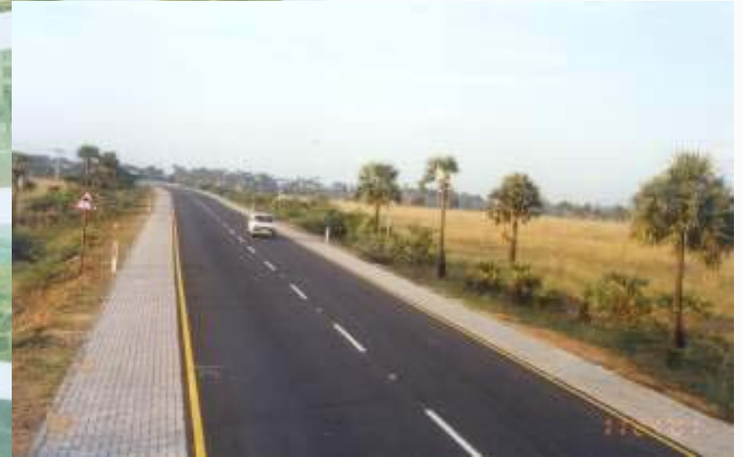
Paving block shoulders where widening not possible due to environmental restrictions (Mahabalipuram to Palar)
