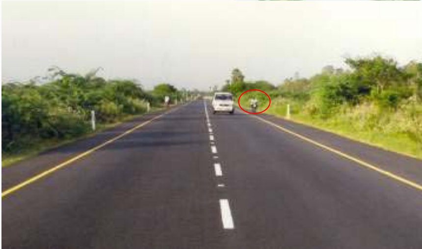
Paved Shoulder of 1.75m used by two wheelers and slow moving vehicles (Chennai to Mahabalipuram)
