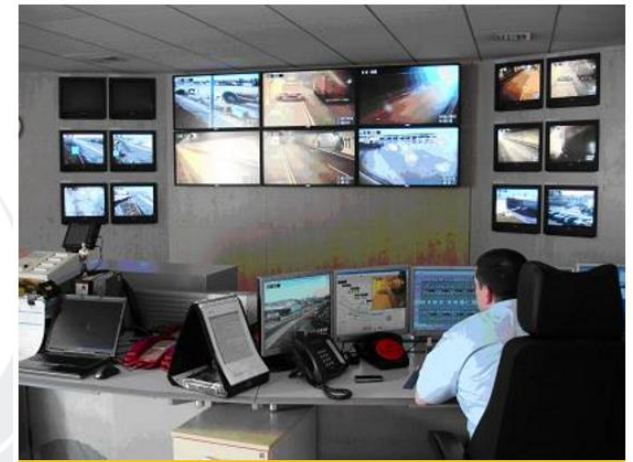
Fig. 3.2-1: Road tunnel command post
