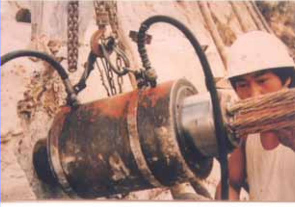
The prestressed anchor cable's extension tonnage are 100t, 160t, 300t and 600t.
